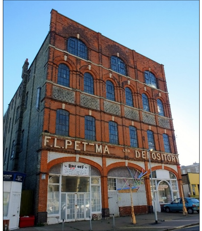
Pettman's Depository building dominates to southern end of Athelstan Road. The decorative design of the front of this building and the use of red bricks contribute towards its appeal. This building, in particular, has much potential to enhance the proposed conservation area. Certainly, it would be good to see the original sign restored!
