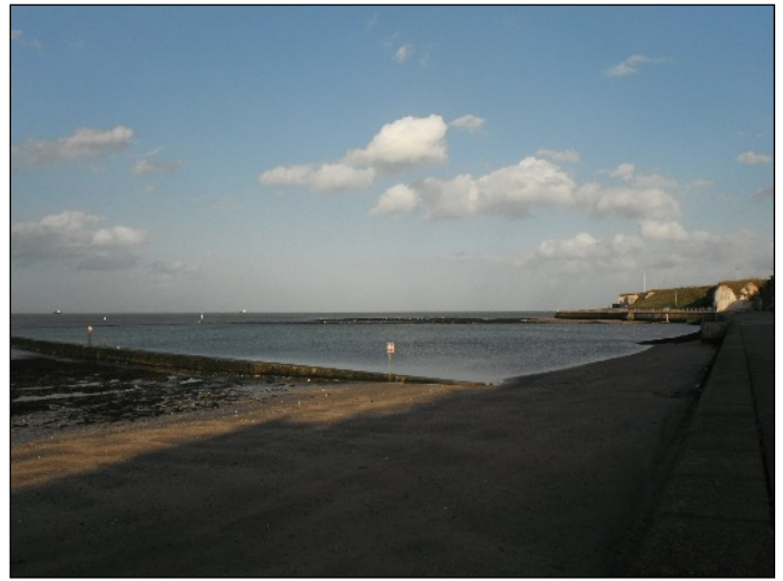
Two photographs showing Walpole Bay Tidal Pool as it is today. In the lower picture, two boys fishing can just be seen at the far end of the wall on the left of the picture. This tidal pool at over four acres is huge: its construction in 1937 by Margate Corporation's direct labour force was rightly considered to be an engineering feat
