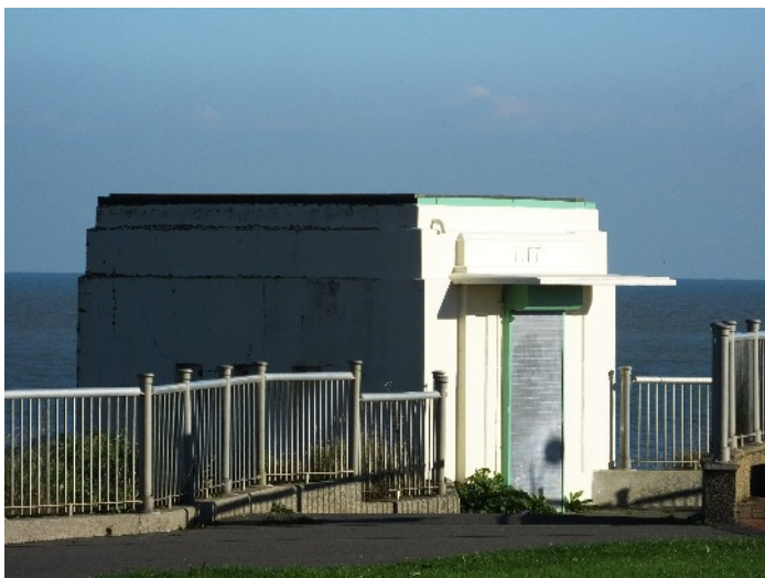
Showing the shutters to secure the building and many weeds which have taken root at the foot of the doorway
