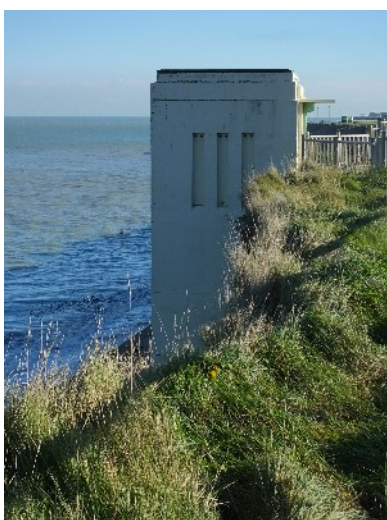
Looking east. The pairs of circular openings seen in each of the three recessed areas are for ventilation purposes
