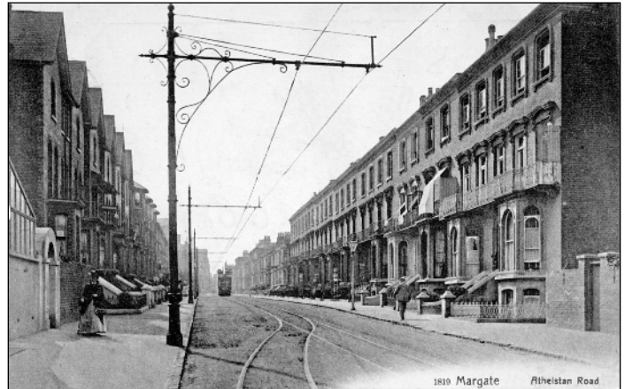
The view from the Ethelbert Terrace end of the road
