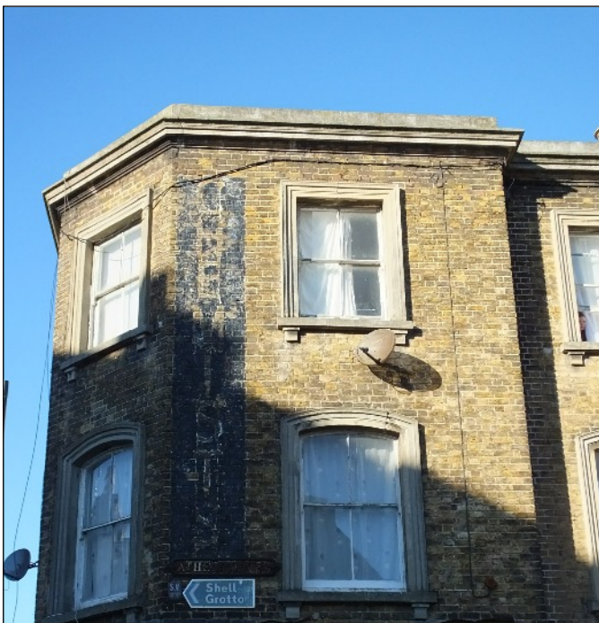
The first and second floors of the former chemist's shop on the corner of Athelstan Road and Northdown Road. The word CHEMISTS can still be read painted vertically on the brickwork of the building. Also, above the modern sign pointing to the Shell Grotto can still be seen the original street name-plate for Athelstan Road
