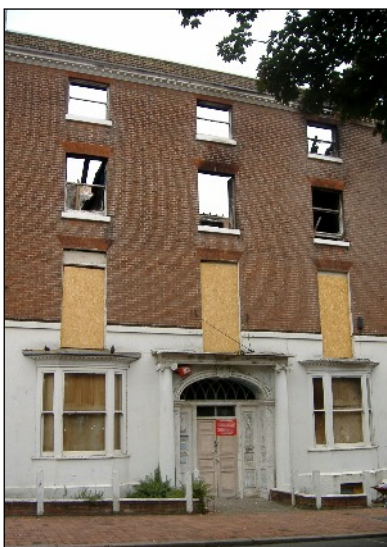
49/50 Hawley Square (now one property) photographed after the fire in 2008 when the roof was destroyed
